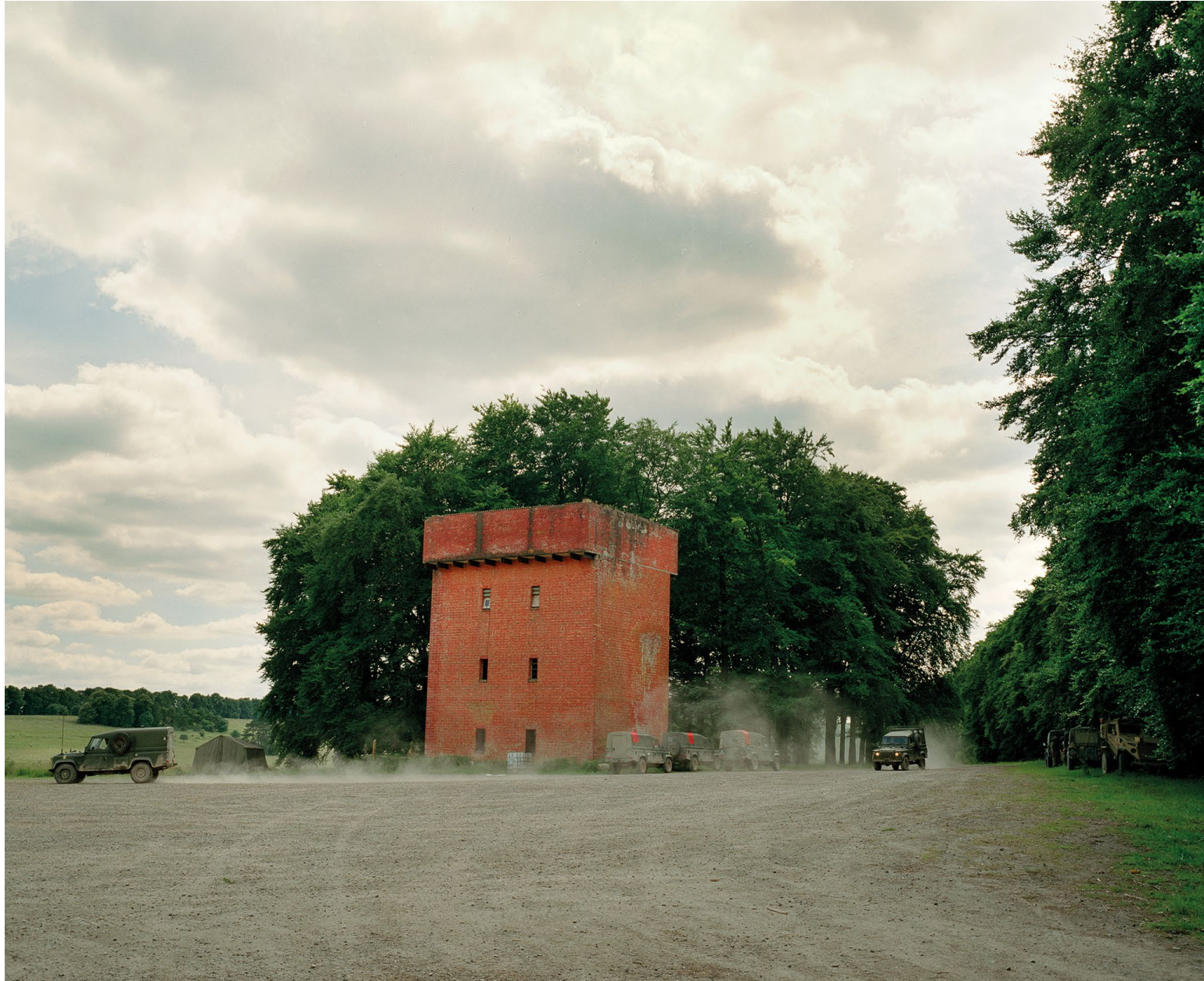
The Water Tower, Tilshead Down. July 2016.
