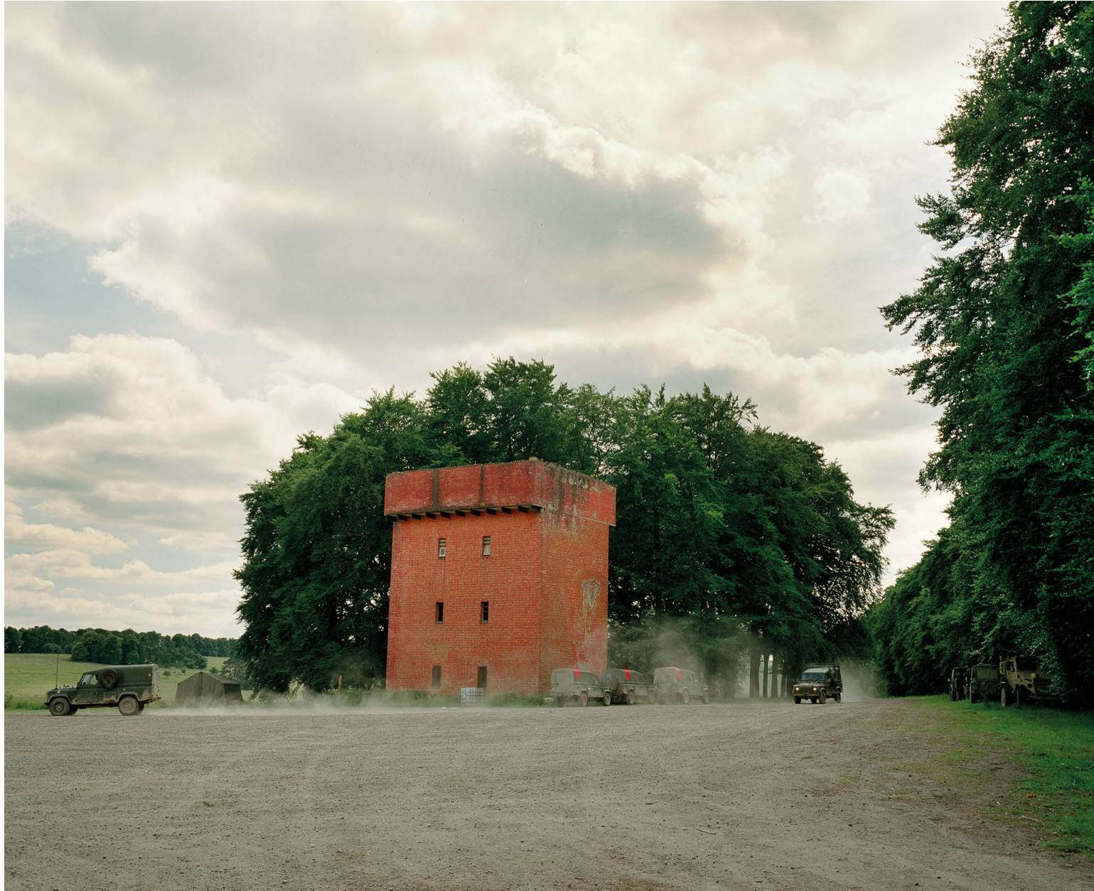
The Water Tower, Tilshead Down. July 2016.
